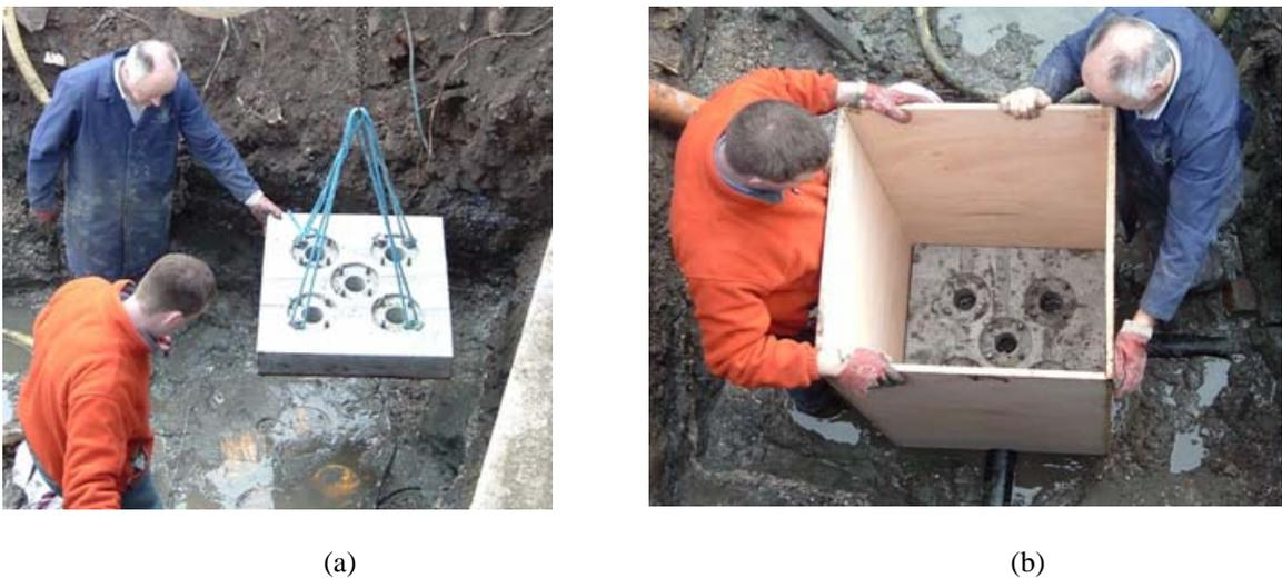
**Fig. 1:** (a) Installation of pre-cast reinforced concrete raft foundation with voids for piles, (b) placement of box to backfill around the raft
