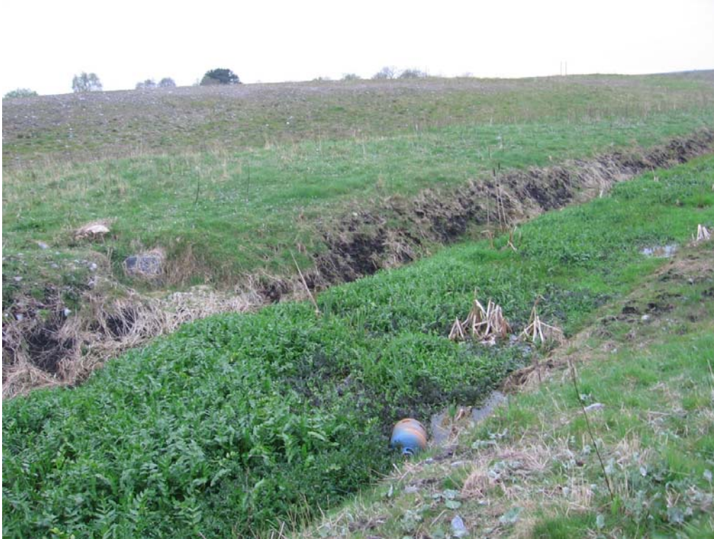
Figure 6 – Clogged stream diversion shown at front and peat disposal area in background at Pollboy 3 years after construction
