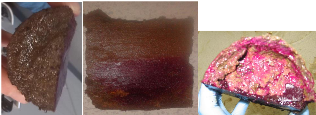
Figure 5.3 - (a) No colour change on top surface of a4(1c) (b) Carbonation depth profile for a5(3c) (c) Pink region on top of surface of B5(1)
