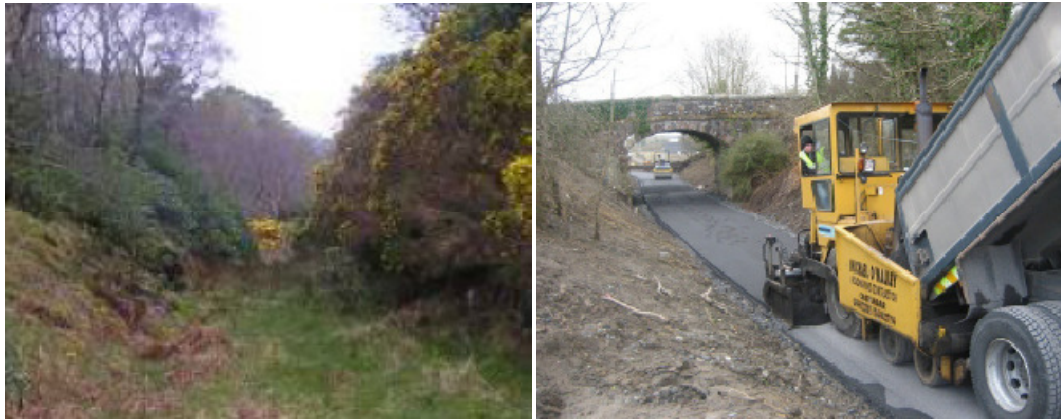
Figure 6.2 - Railway trackbed (left) and GWG construction (right) (Connor, 2013)
