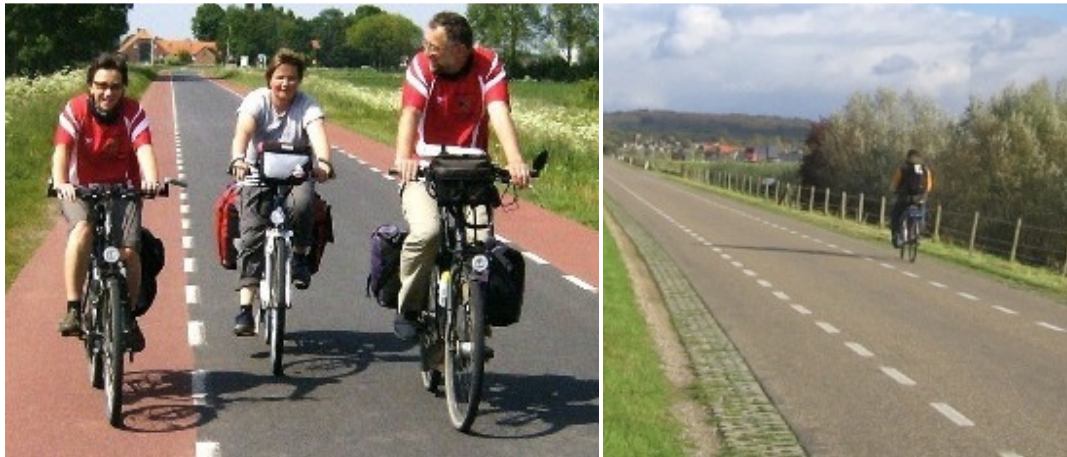
Figure 8.9 - Advisory cycle lanes on EV2: D-Netz 3, Saxony-Anhalt, Germany (left) (Anhalt-Dessau-Wittenberg, 2015) and LF4, South Holland, Netherlands (right) (ECF, 2015)
