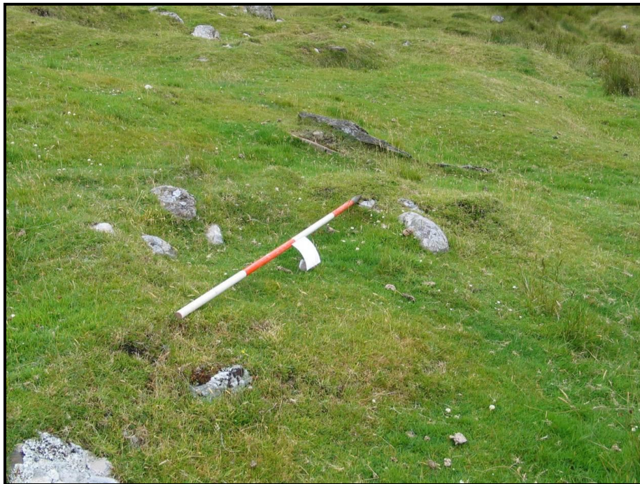
Pl. 90 - The low foundations of House I at Keem Village - all that remains today!
