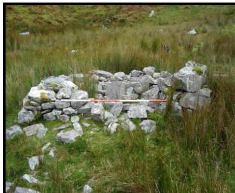
Pl. 61 – House 8 at Bolinglanna (Bol8) showing the partition wall and fallen masonry within the house.
