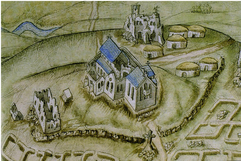
Fig. 28 – The Creat, a sub-rectangular structure, with rounded ends, supported on cruck trusses that lay directly on the ground (after Hayes-McCoy 1964, 8).
