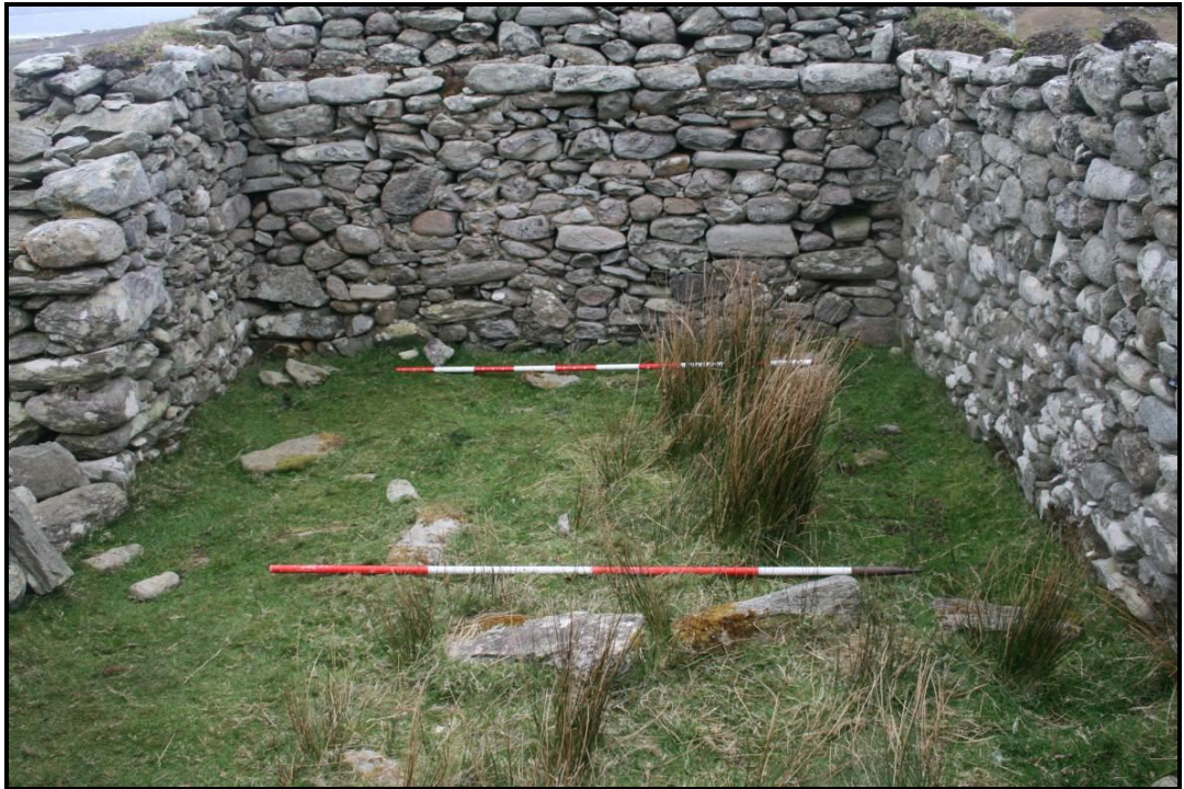
Pl. 43 – Remains of the stone ridge of an overhead loft on internal south gable wall at House 19 (S19) at Slievemore.
