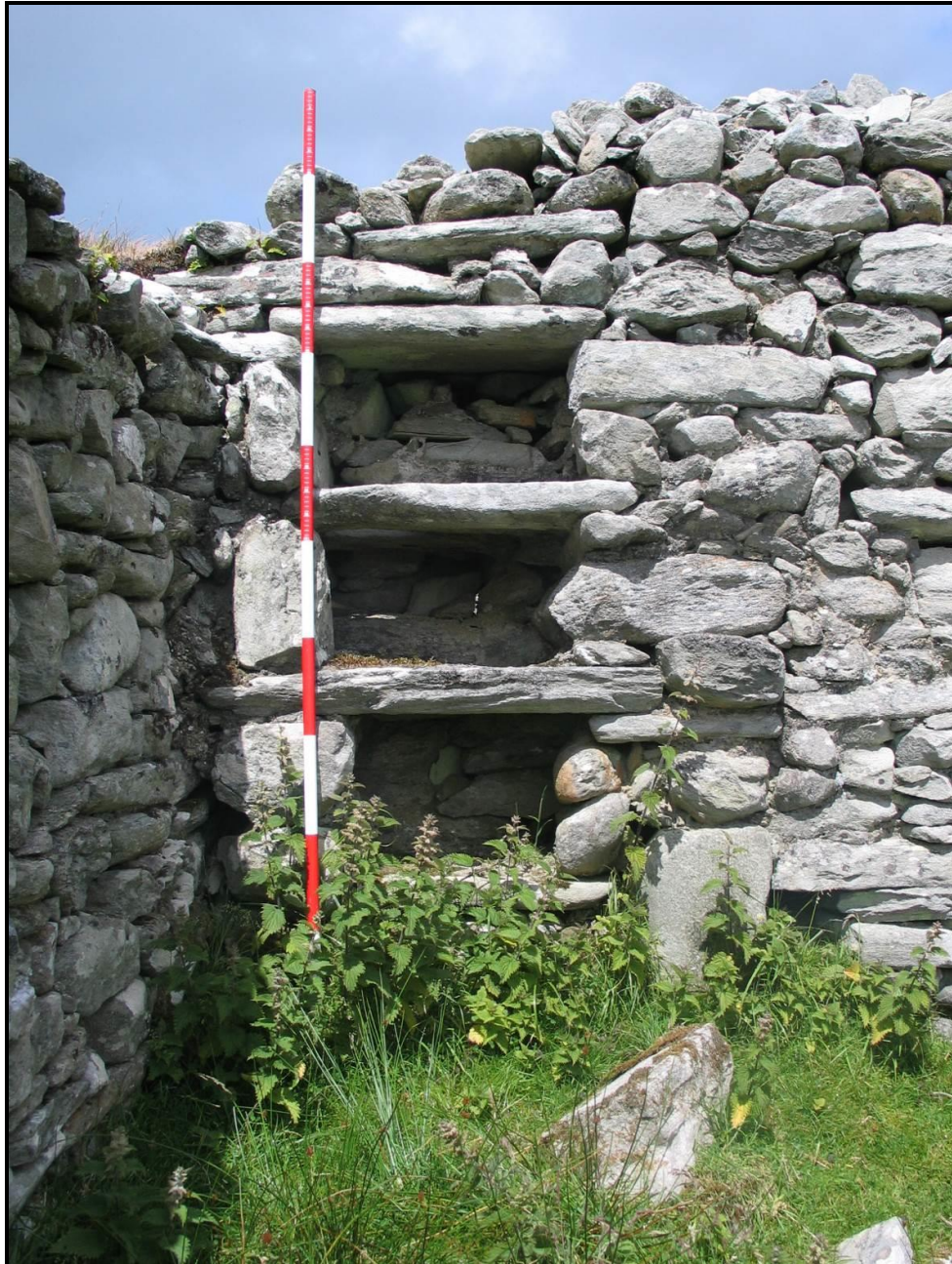
Pl. 93 – Three storage niches, one above the other, in House 13 (S13) at Slievemore.
