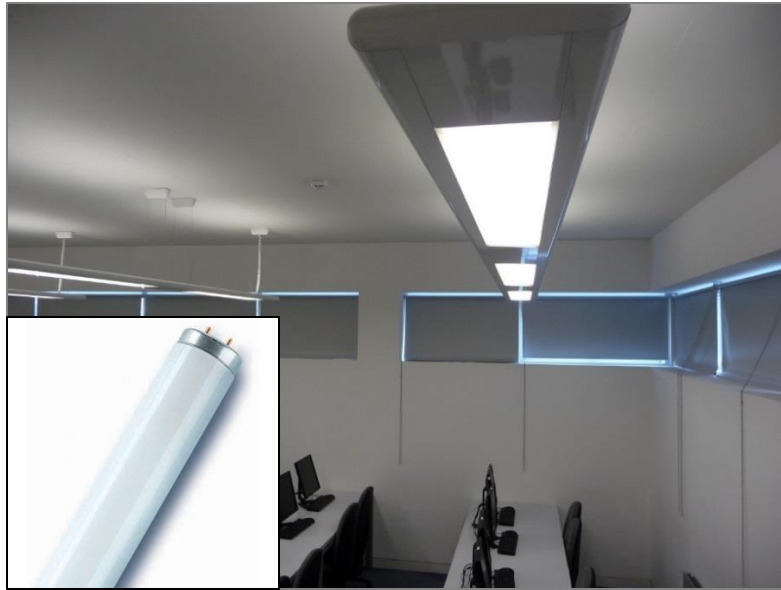
Figure 4-19: Typical lighting fixture and close-up of T8 fittings (inset)
