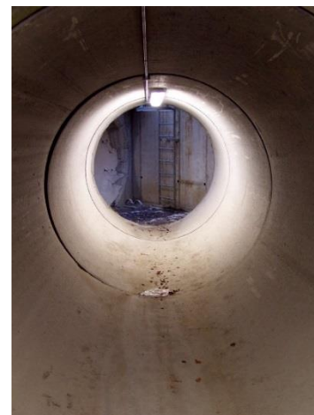
Figure 4-2: Earth Tube / Earth-Air Heat Exchanger
