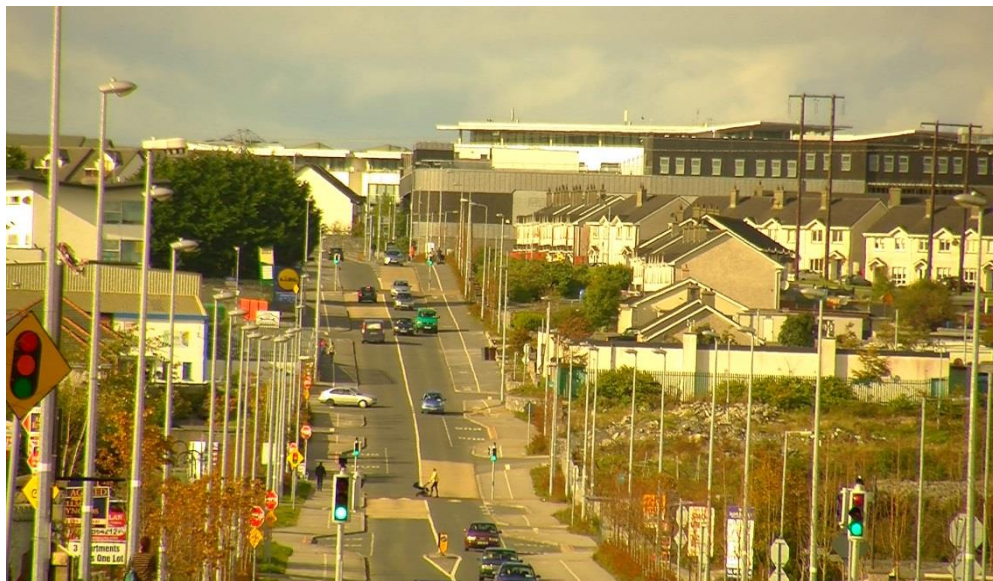
Figure 19 - The new Doughiska Road.
