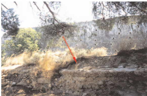
Fig. 5. The Roman aqueduct channel is indicated by the arrow in the foreground while the high substructure wall is that of the Egyptian aqueduct.
