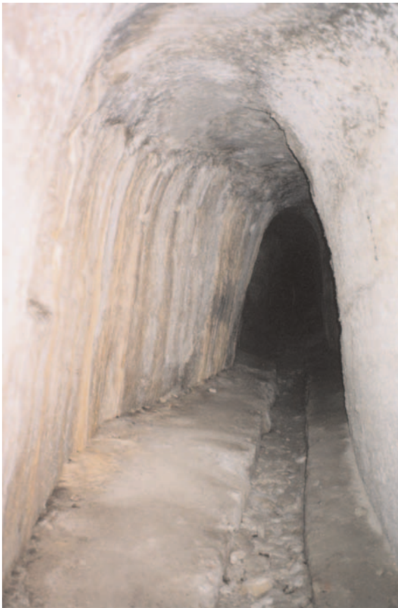
Fig. 6. The aqueduct at Eleutherna.
