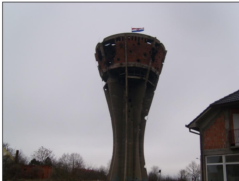
Image 5.20: Vukovar Water Tower, 2009 The tower is preserved in its war damaged condition post 1991
