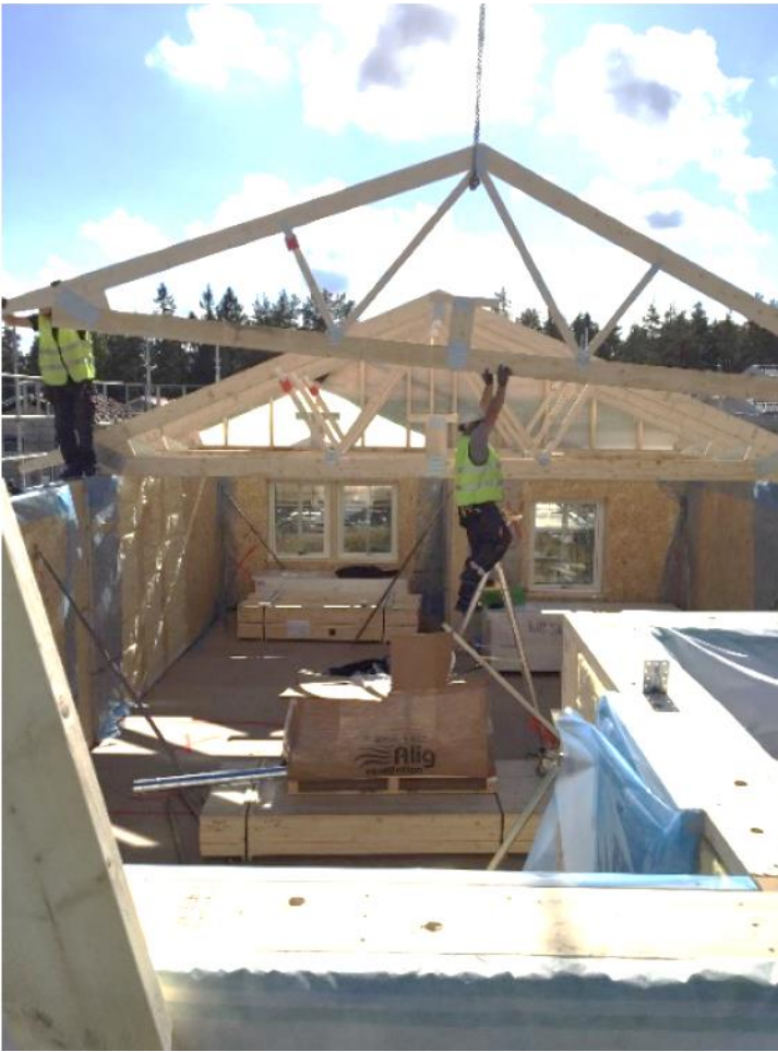
Figure 2-12: Derome roof truss lifted into position on site (image courtesy of Derome)
