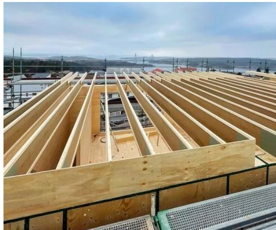
Figure 3-2: Mass timber panels for walls and intermediate floor(left); I-joist roof structure (right).
