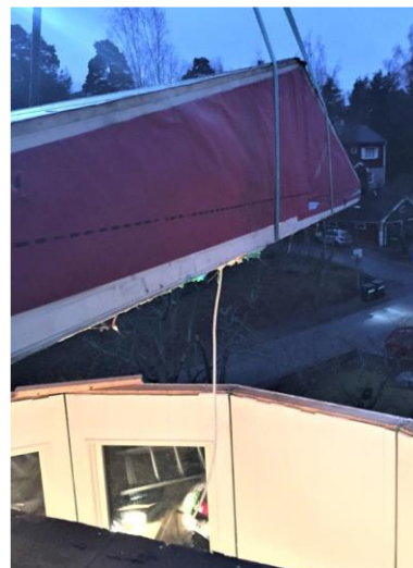
Figure 3-5: Magnolia Pavilion roof cassette reassembled in Segeltorp, Sweden (image courtesy of IsoTimber).
