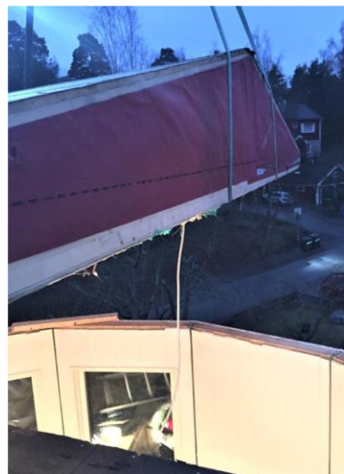
Figure 3-5: Magnolia Pavilion roof reassembled in Segeltorp, Sweden (image courtesy of IsoTimber).
