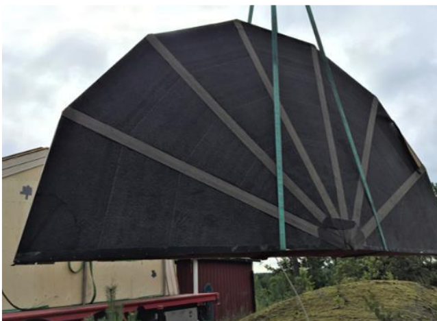
Figure 3-4: Magnolia Pavilion roof cassette demounted for transport in Tyresö, Sweden (image courtesy of IsoTimber).
