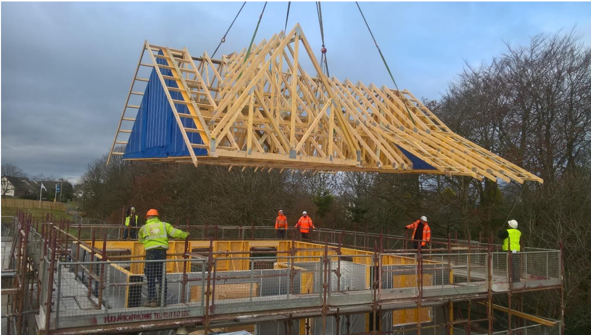
Figure 2-23: House roof structure lifted into position on Robertson site
