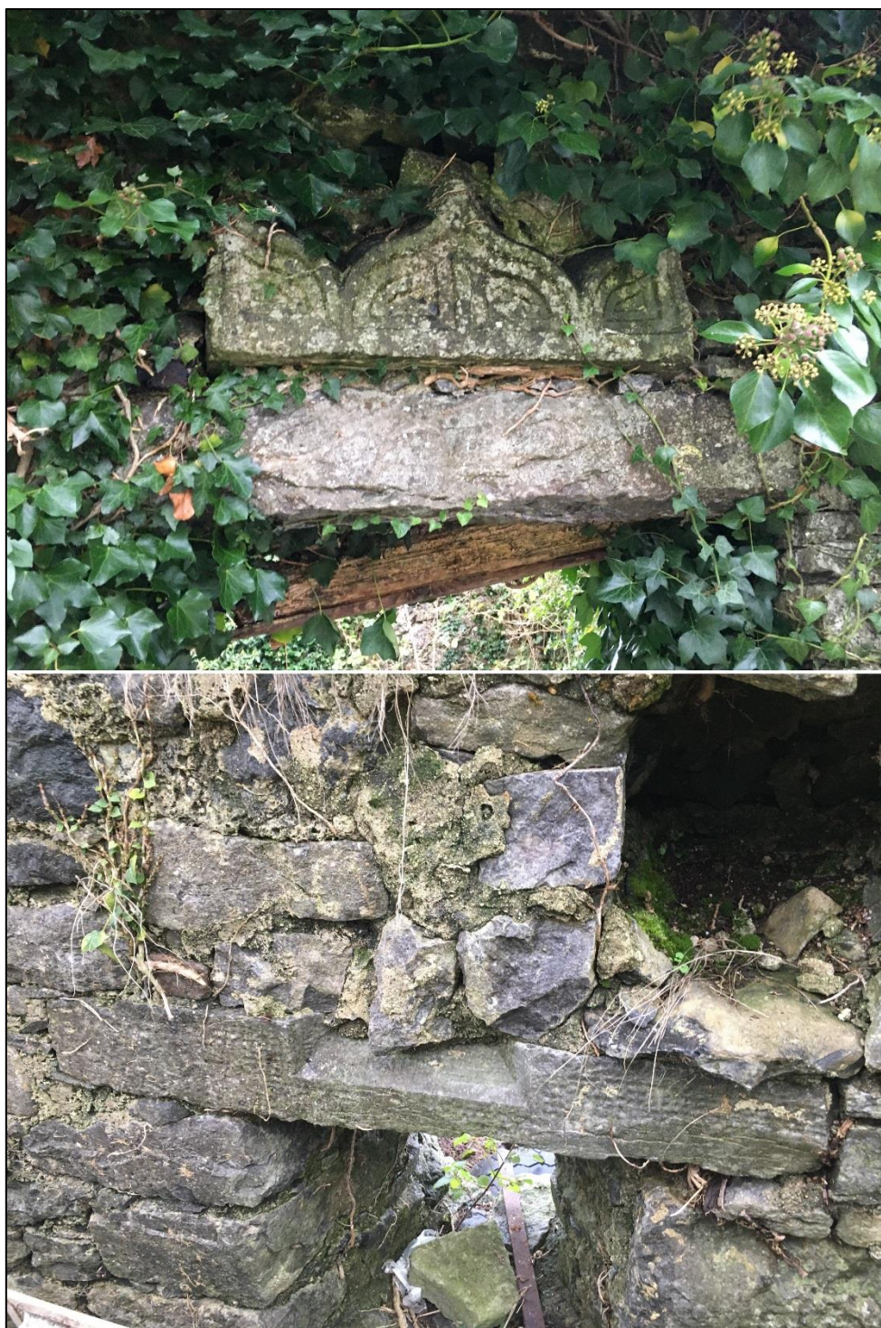
Plate 7.5 - The upper [top image] and lower [bottom image] sections of a two-light ogee-headed window, incorporated into an outbuilding adjacent to Sandfield House, and presumably recovered from Lisdaulan Castle (Author's photographs).
