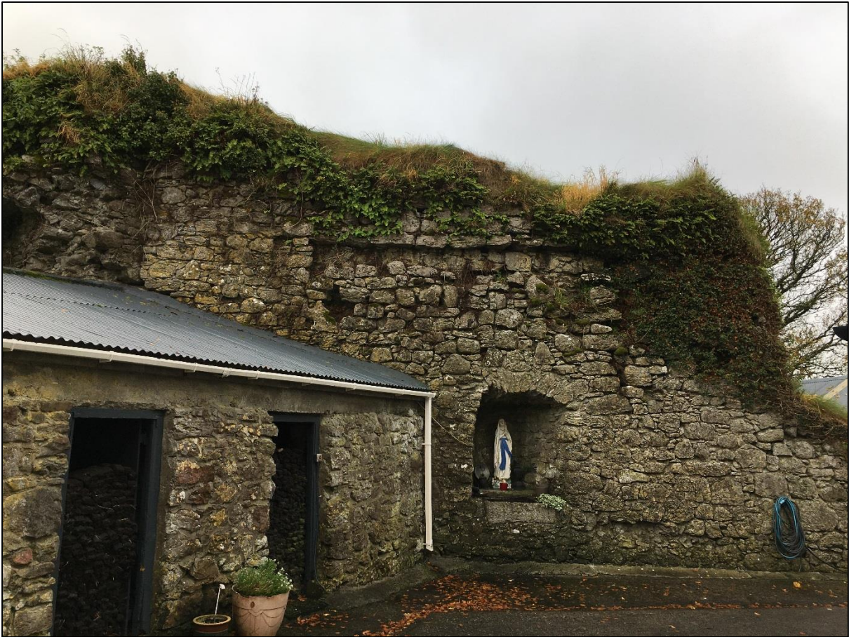
Plate 5.8 - Interior view of much modified castle wall at Callow Castle. The lance window [centre of image] has been blocked up and turned into a grotto, and the first floor joist holes and ceiling recess is evident above it. (Author's photograph)
