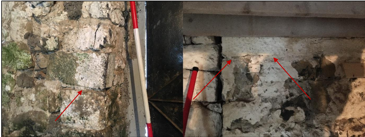
Plate 5.1 - Some examples of the range of punch-dressed stones, indicated by the red arrows, which have been incorporated into the building fabric of an outbuilding attached to Turrock House (Author's photographs).
