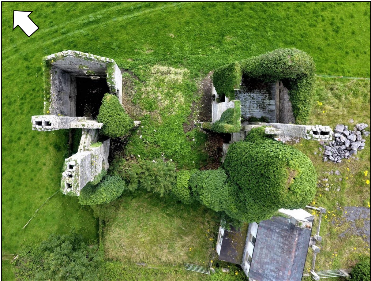
Plate 6.9 – Vertical aerial image of the fortified house now known as Athleague Castle. The two projecting towers flank a ruined rectangular building, which was located centrally on the image, between the pair of chimney stacks oriented northeast/southwest. North indicated by the white arrow. (Image courtesy of Carl Bryer)
