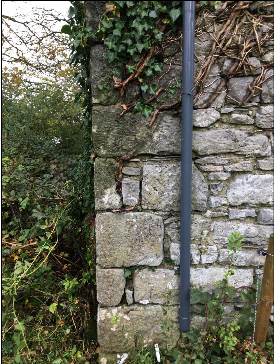
Plate 5.9 - One example of the finely tooled punch dressing to be found incorporated into the fabric of the modern farm buildings on the site of Callow Castle (Author's photograph).
