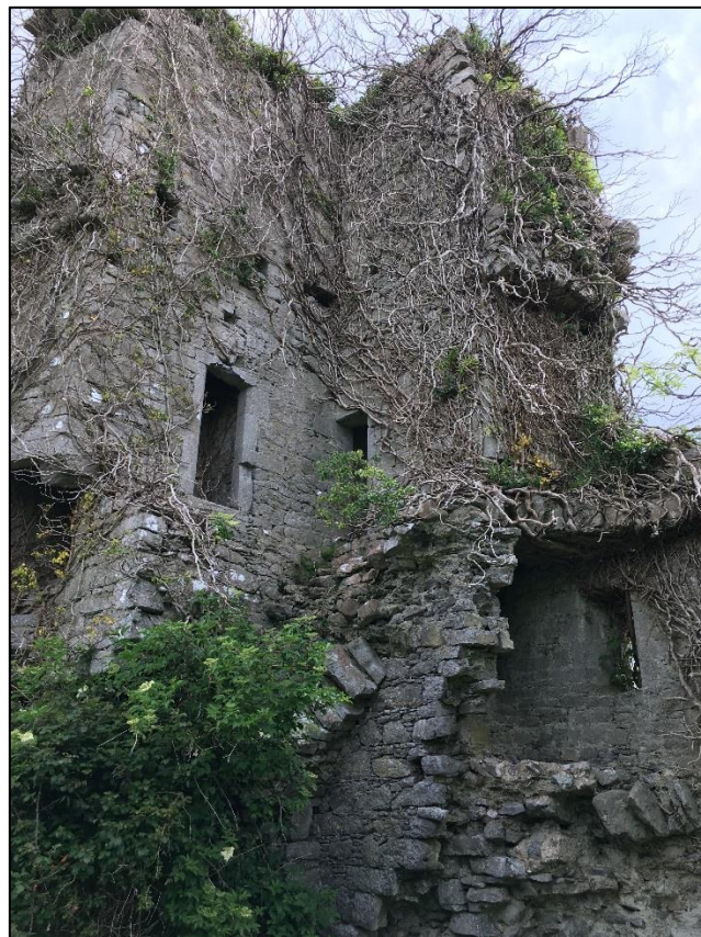
Plate 6.5 – Ground image of the internal remains in Gale tower house, viewed from the southwest. Note the vaulting in the centre foreground of the image, the window and intramural stairway in the right foreground, linking the first floor to the second floor. Access to the third floor, and joist holes for the third floor platform is visible to the top of the image (Author’s photograph).
