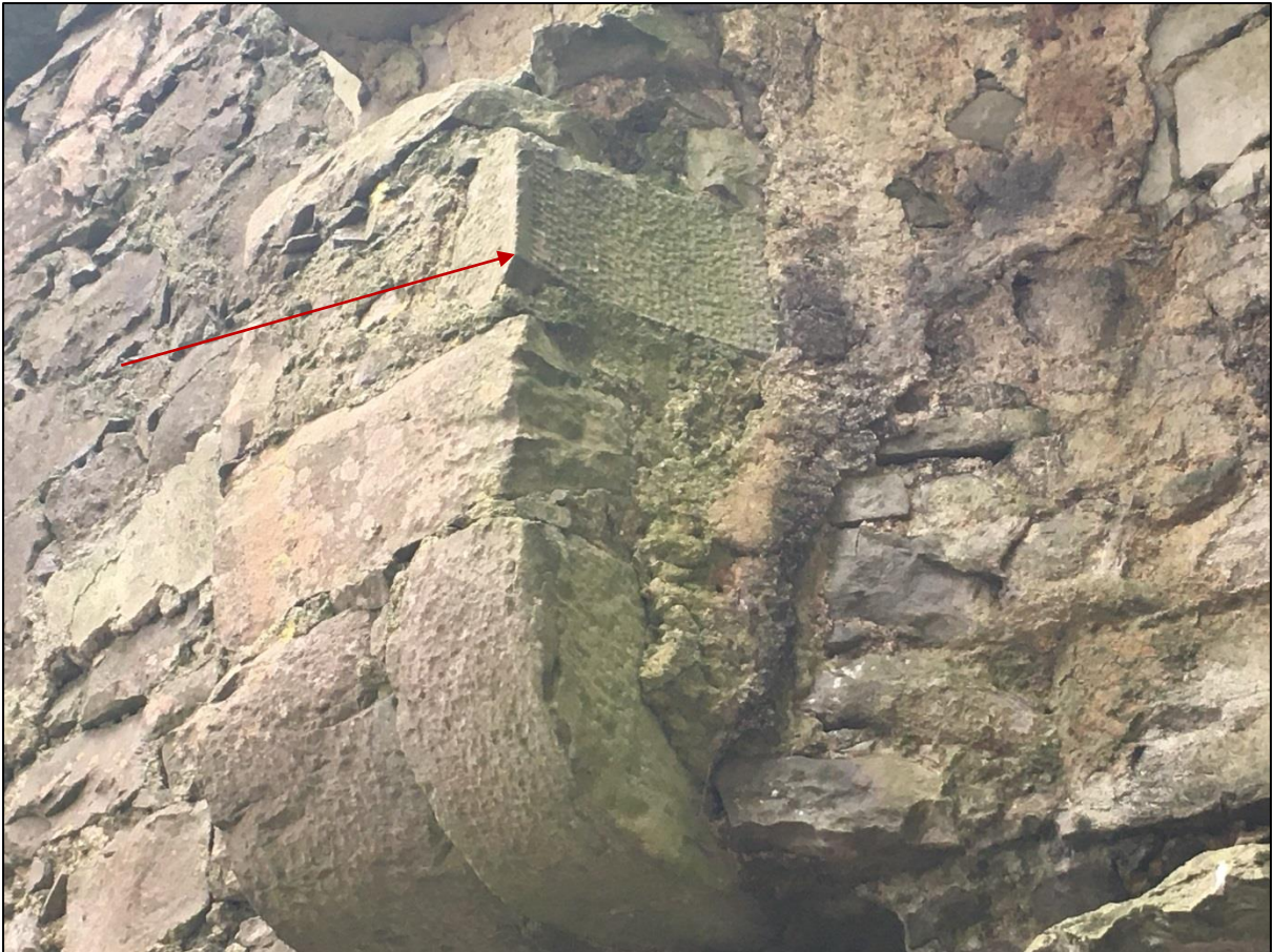
Plate 6.10 – One example of the punch-dressed stone from within the fortified house of Athleague Castle. This cut stone was one of two such pieces incorporated into a first floor fireplace in the north-western flanking tower of the castle (Author's photograph).
