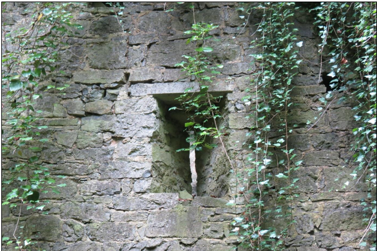
Plate 6.012 – The best preserved of the loops which are incorporated into the building fabric of a mill building located in Mote Demesne, Co. Roscommon. This is possible evidence for the remodelling of the mill building out of the remains of a tower house castle. (Image courtesy of Martin A. Timoney).
