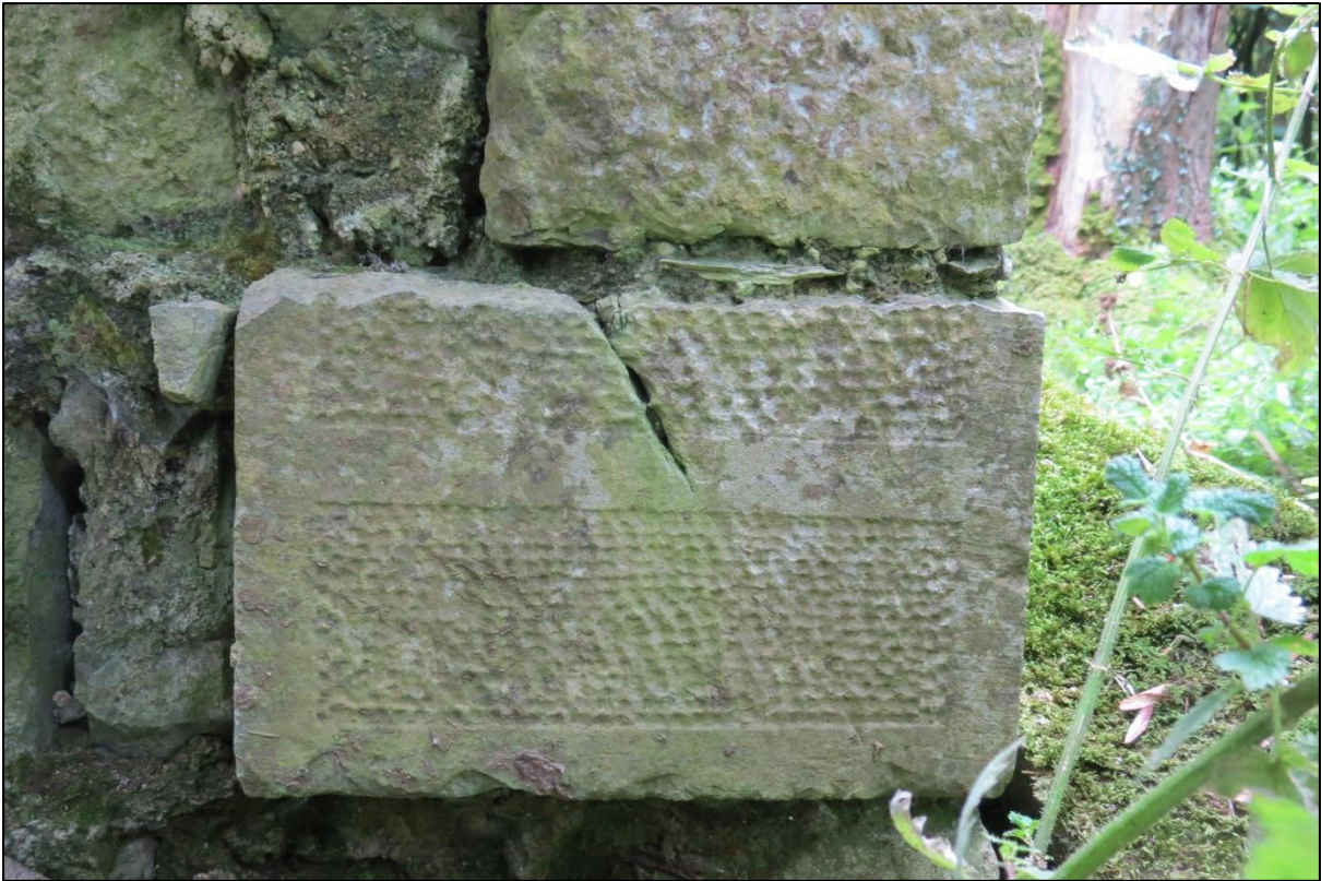
Plate 6.013 – One of the finest examples of punch-dressing found incorporated into the mill building in Mote Demesne, Co. Roscommon, which leads to the conclusion that the historically-attested Ó Cellaig castle at Mote was located here, and is likely to have taken the form of a tower house (Image courtesy of Martin A. Timoney).
