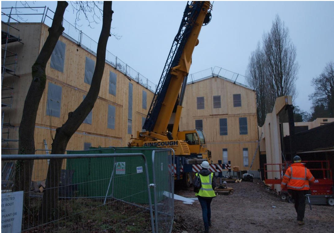
Figure 5.32 CLT construction in Bishop's Stortford, UK: Test building
