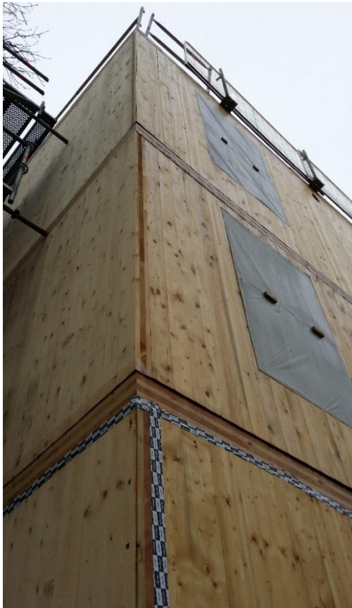
Figure 2.10 CLT platform construction
