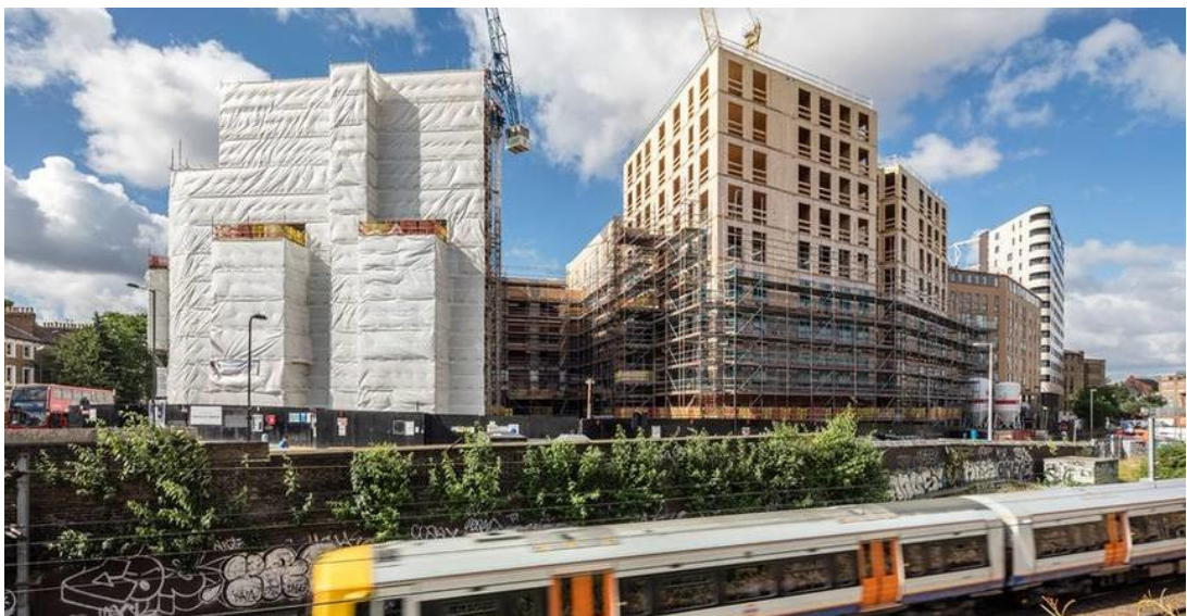
Figure 2.4 Dalston Lane adjacent a high-speed railway line [Image by Daniel Shearing [38]]
