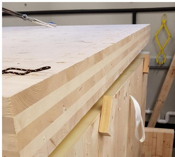
Figure 5.19 Assembly C during construction
