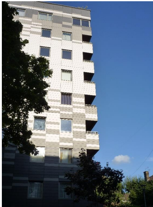
Figure 2.2 Murray Grove, a nine-storey residential building in Hackney, London, 2009
