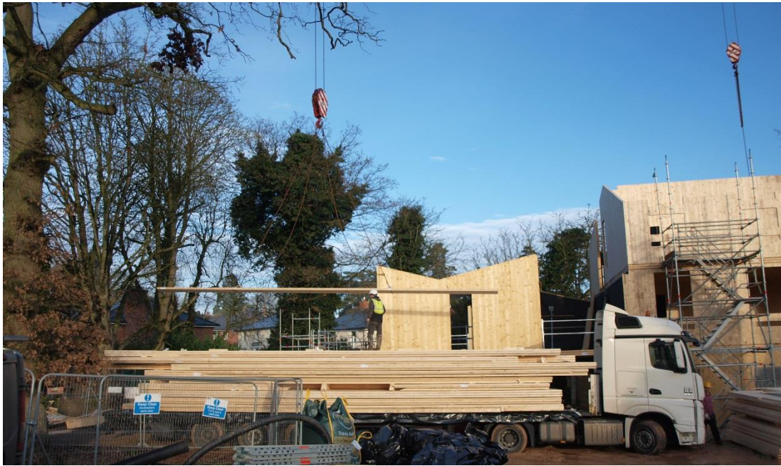
Figure 5.33 CLT construction in Bishop's Stortford, UK
