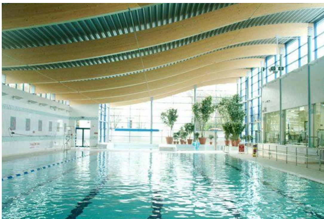
Figure 1.1 Glulam roof structure: Ballinasloe swimming pool [5]
