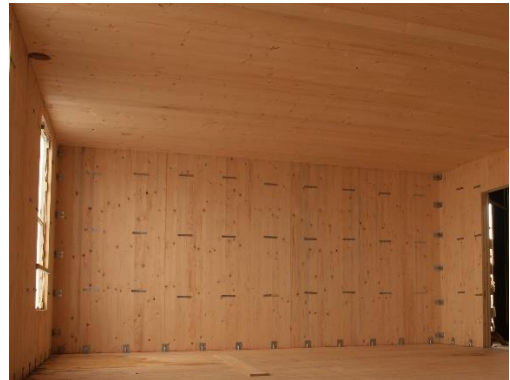
Figure 2.11 CLT platform construction
