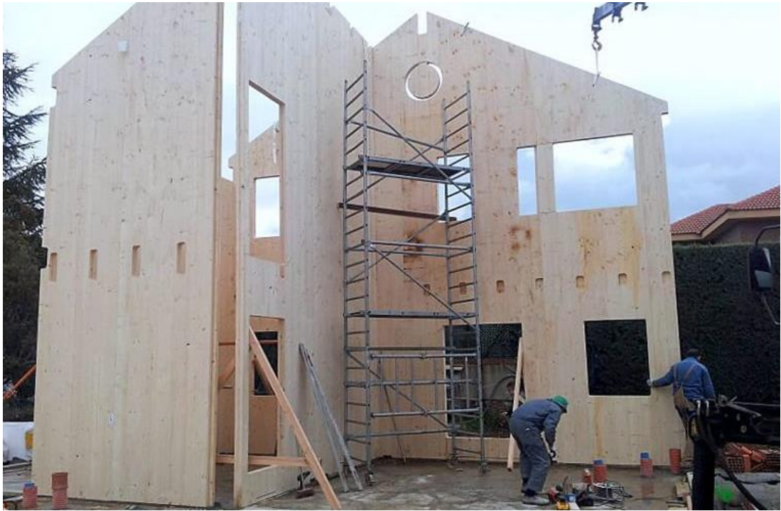
Figure 2.9 CLT balloon construction [Image by GB-Legname [51]]
