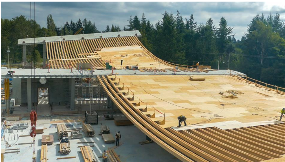
Figure 1.4 Grandview heights aquatic centre, under construction [Image by Seagate Mass Timber [8]]
