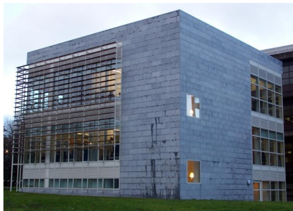
Figure 2. Nursing Library building at the National University of Ireland Galway.
