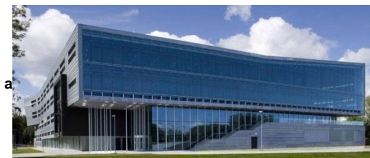
Figure 2. Engineering Building at the NUI Galway (a) and modelled meeting room (b).
