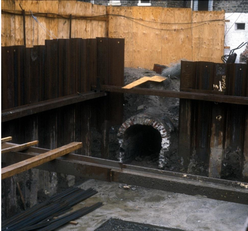
Figure 4.8 Culverted section of the Swan River, Mount Pleasant Avenue, Dublin, 1986 (Author: Patrick Healy, Source: South Dublin County Council)
