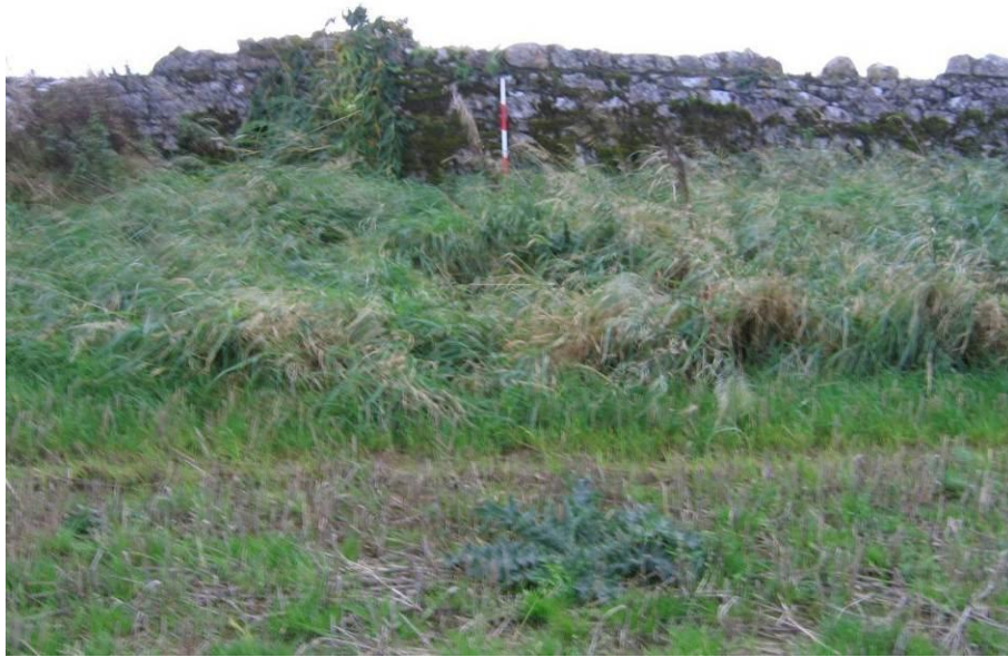
Pl. A7.6: 1.3m mortared stone wall on 0.5m bank, D9
