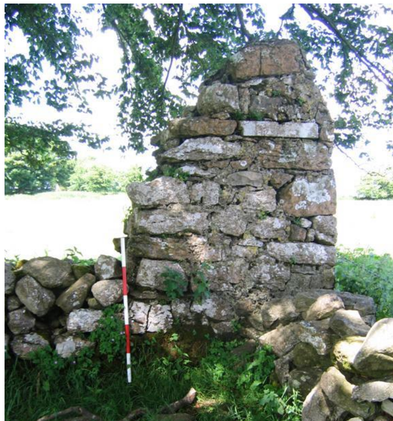
Pl. A5.32: Northern wall end from the south showing re-used cut-stone masonry and repair
