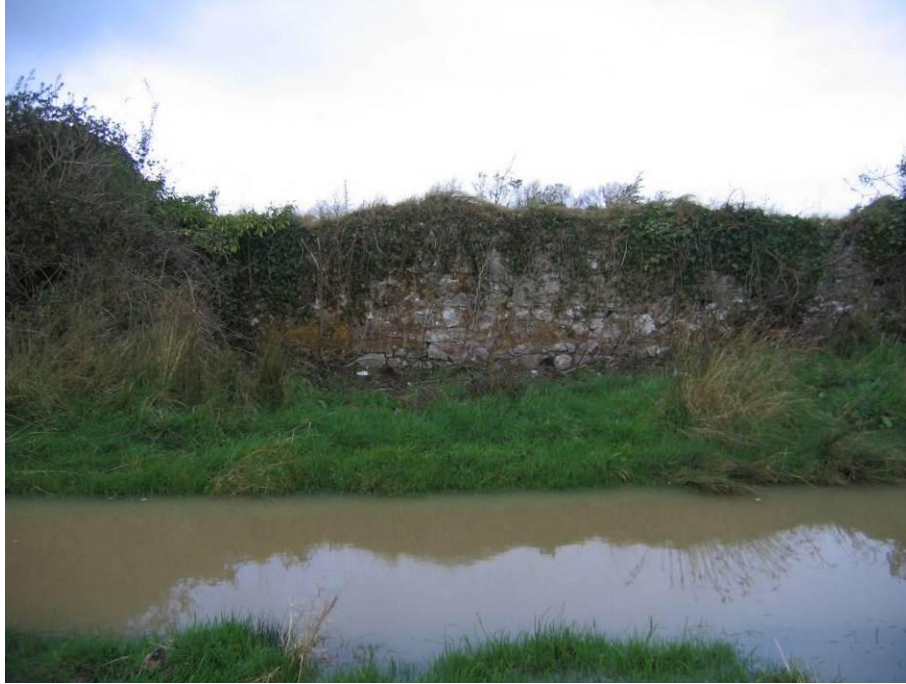
Pl. A7.10: Wall c. 2m high on far side of modern ditch, D21
