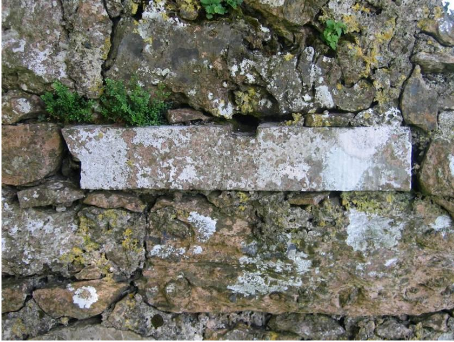
Pl. A5.29: Reused masonry piece
