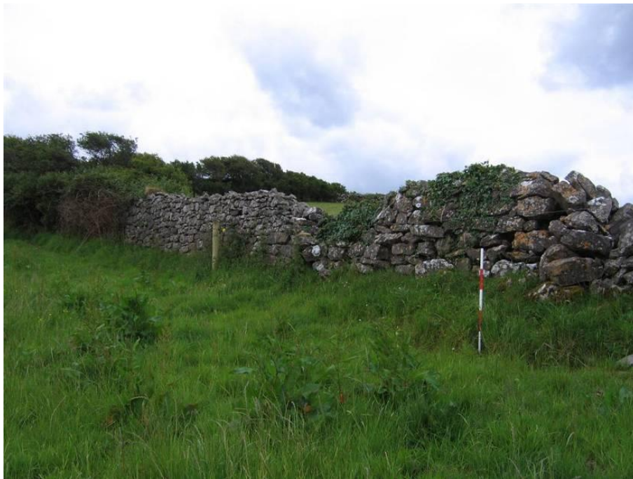
Pl. A5.17: Well preserved wall and 0.5m high bank, E23
