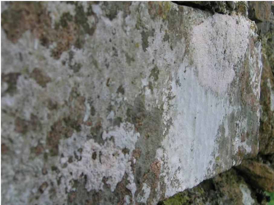
Pl. A5.30: Vertical tooling on the reused masonry piece
