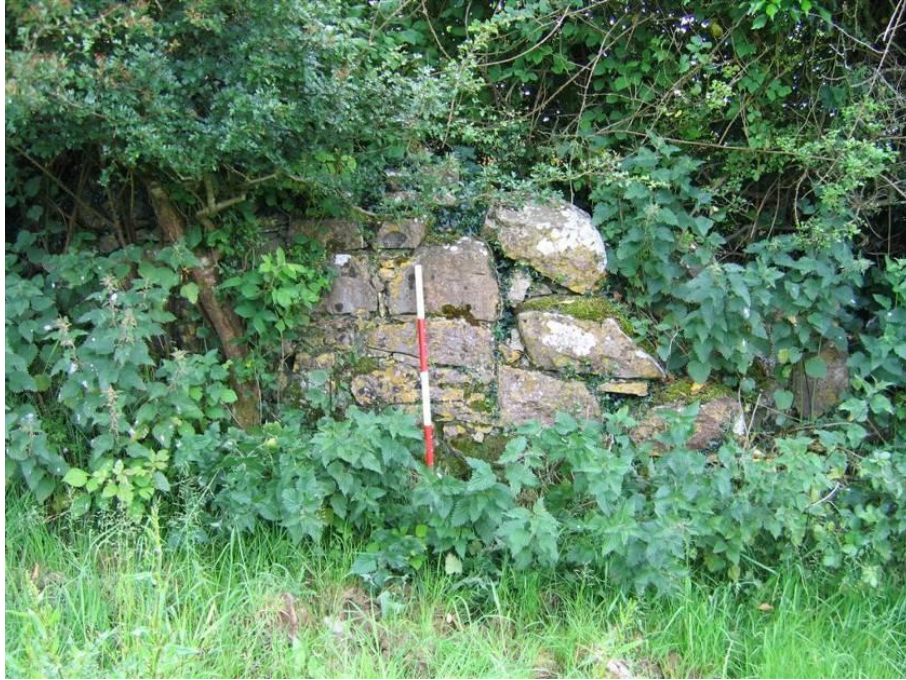
Pl. A5.12: Undergrowth protecting original wall, E16
