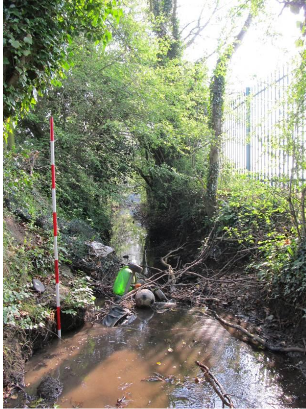
Pl. A6.4: 2m deep, 3.5m wide ditch. Looking southeast. To the right of the picture are the playing fields of NUI Maynooth, while to the left is a modern housing estate, M7
