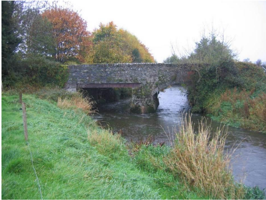
Pl. A9.10: Kyleeragh Bridge and the western riverbank, N14
