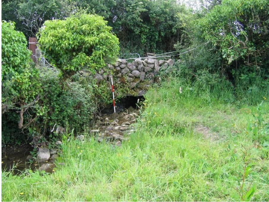
Pl. A5.11: Bridge over the stream, E14
