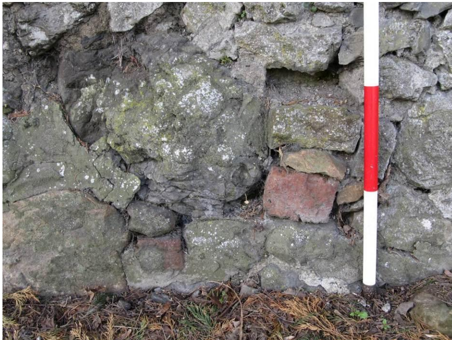
Pl. A9.5: Brick visible in the base of the wall, N9
