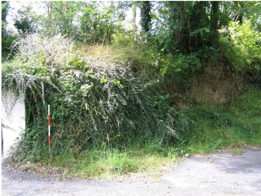
Pl. A5.4: Bank of townland boundary at Killeenadeema road, showing track cut in immediately to the south, E4
