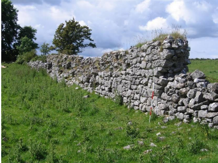
Pl. A5.37: 20m stretch of wall at 2m height, E40
