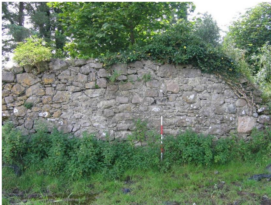
Pl. A5.3: High section of wall close to cattle shed showing up to 2m of probable original wall topped by 0.4m of modern repair at centre, E2
