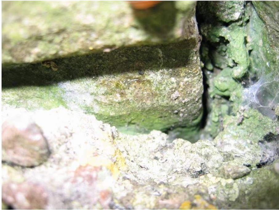
Pl. A5.31: Grooved channel on the reused masonry piece, viewed from below
