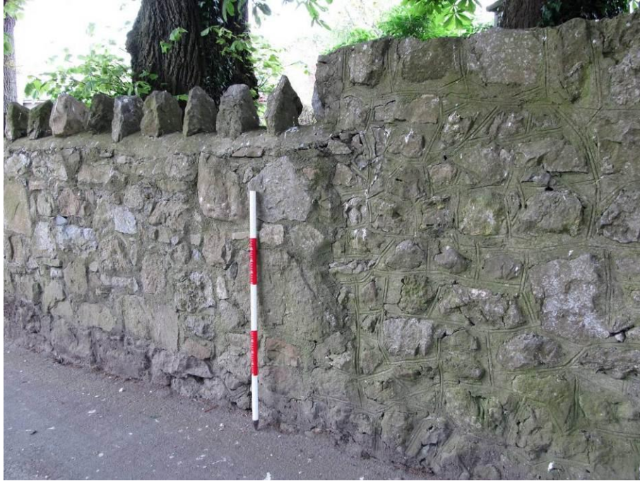
Pl. A9.2: Junction between two phases of wall construction, N3
