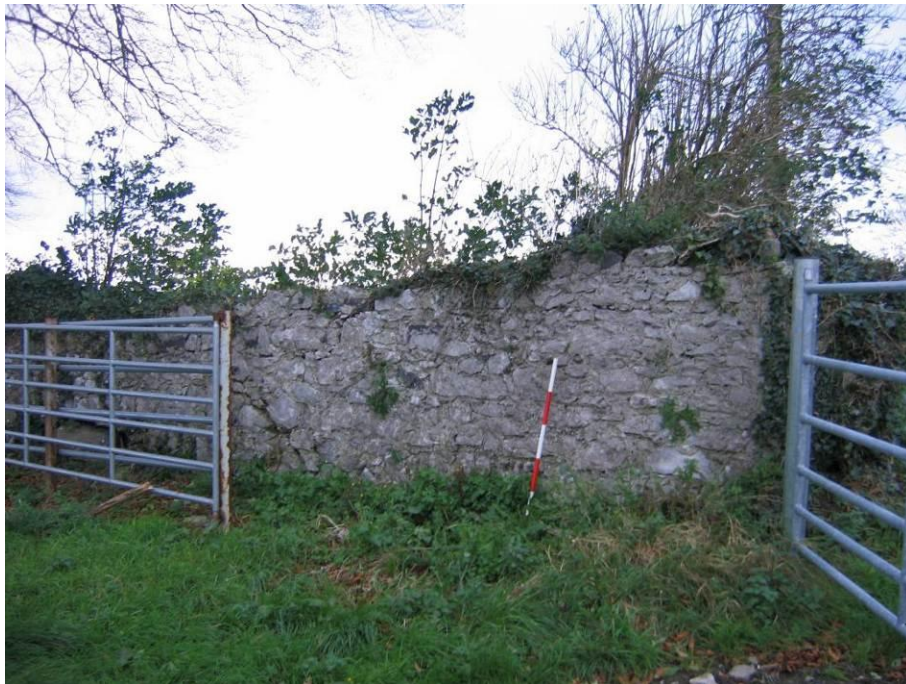
Pl. A7.11: Wall 1.7m high in four phases, D23
