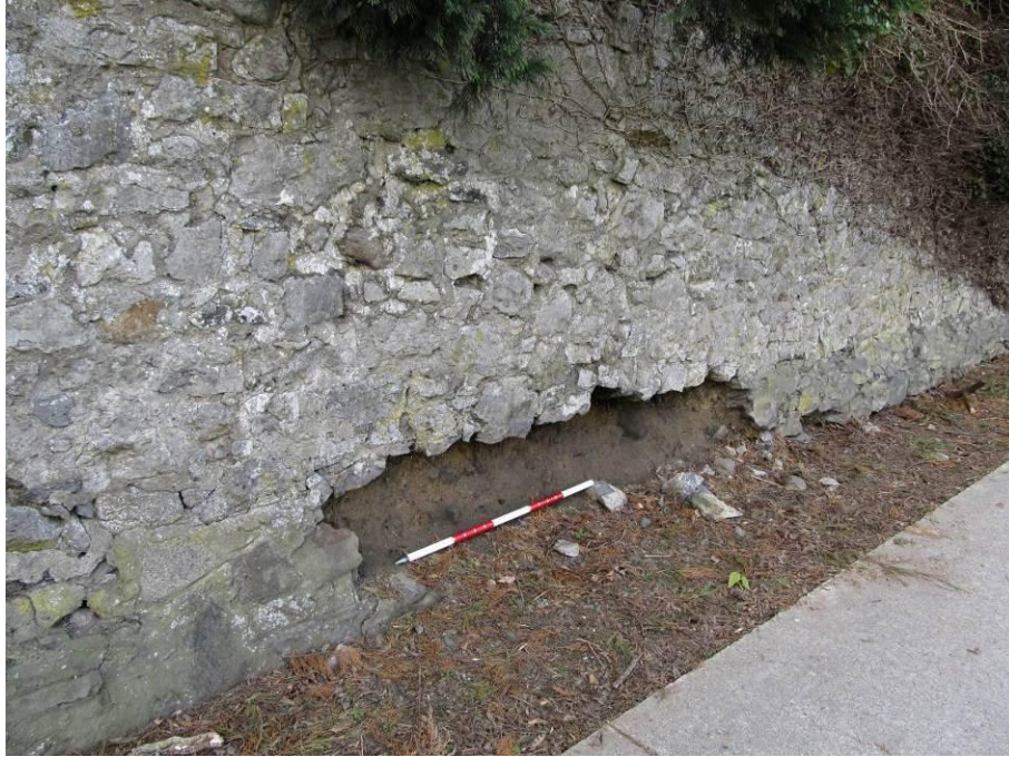
Pl. A9.4: Earthen core exposed at base of wall, N9
