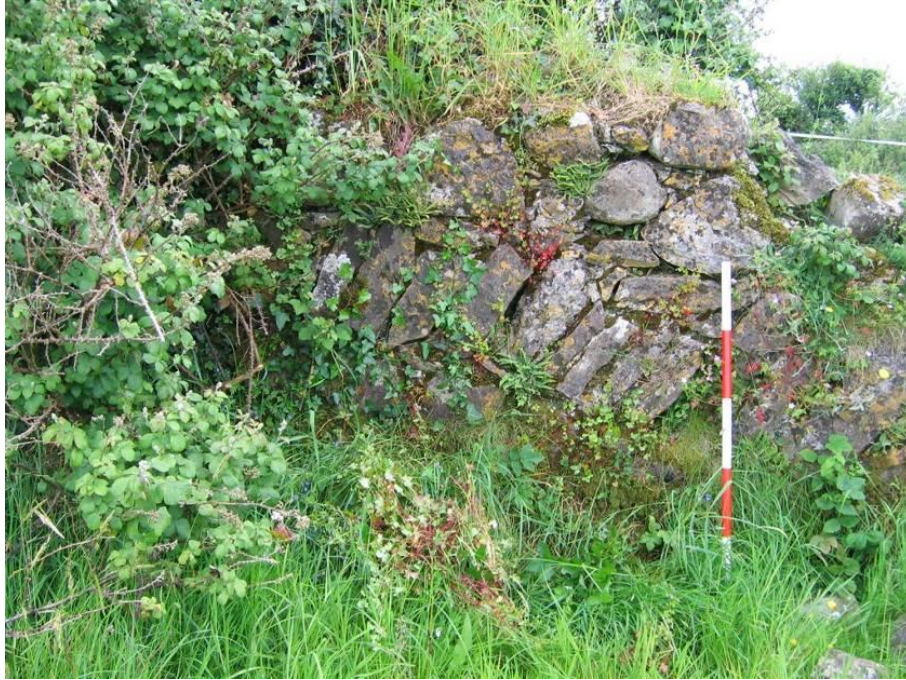
Pl. A5.13: Blocked arch in stonework, E17
