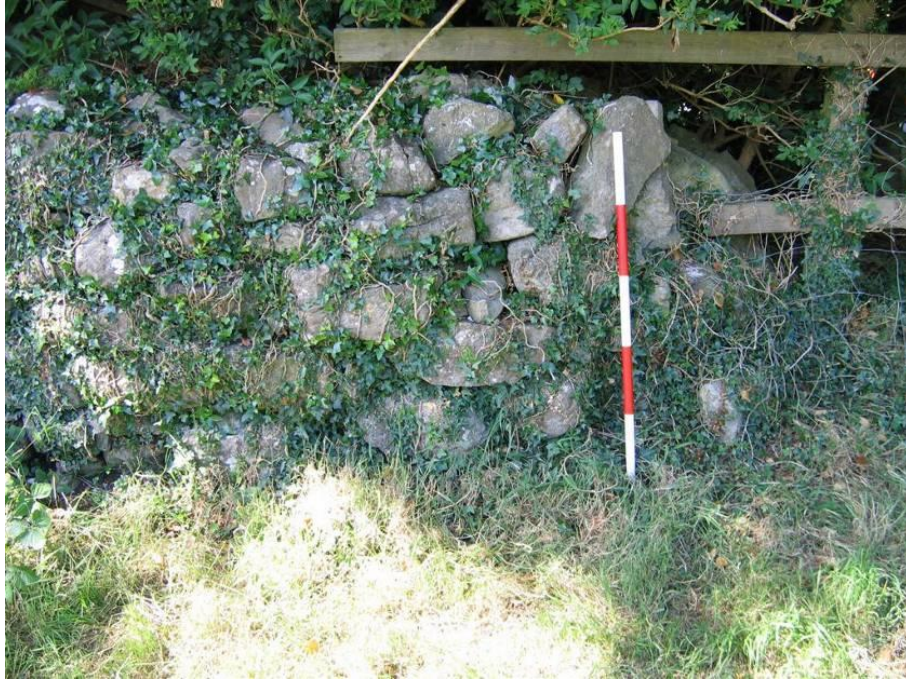
Pl. A5.5: Start of reconstructed wall at end of garden, E6
