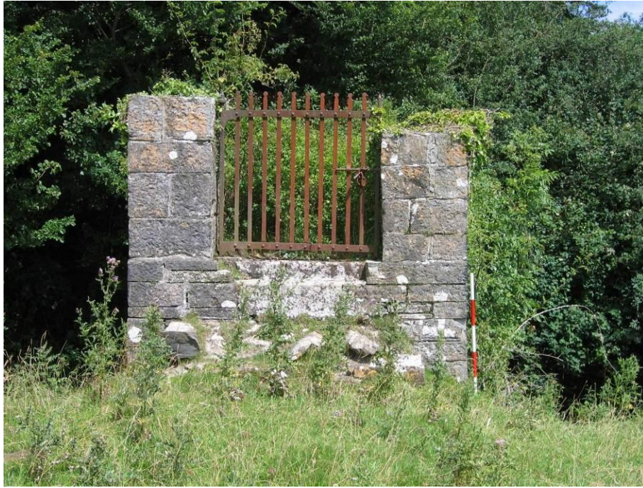
Pl. A6.15: Nineteenth- or early twentieth-century footbridge, M29
