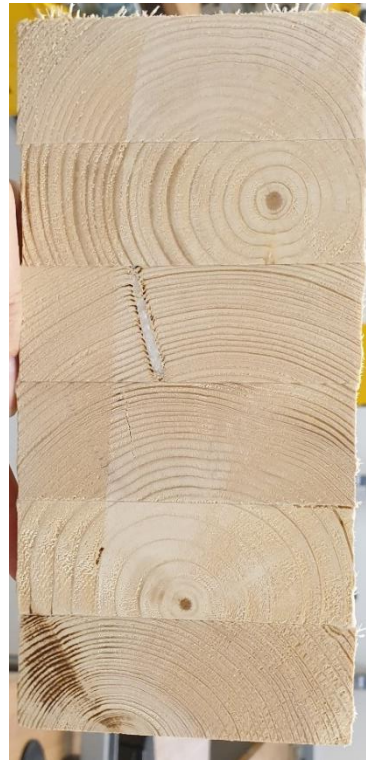
Figure 3-10: Unusual defects can be present in recovered wood, here a screw hole.
