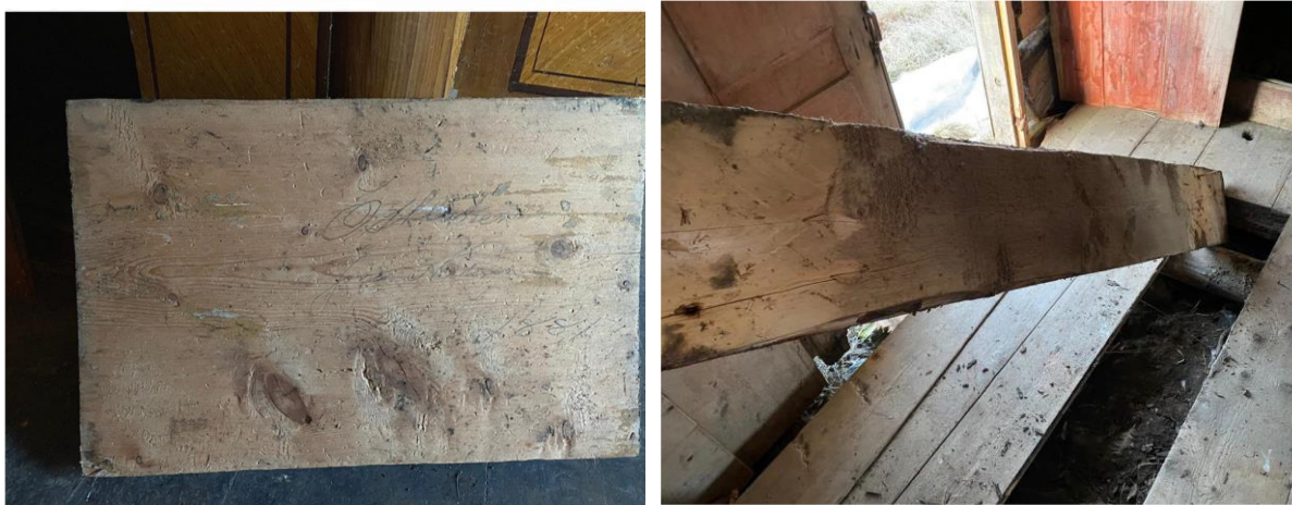
Figure 2-26: To the left: Hand-note written on a piece of the floor: “Östbacken, Jonas Nilsson, 1881”. To the right: recovered timber taken from the floor of the house to be prepared for reuse (photo by Mikael Östling, IsoTimber)
