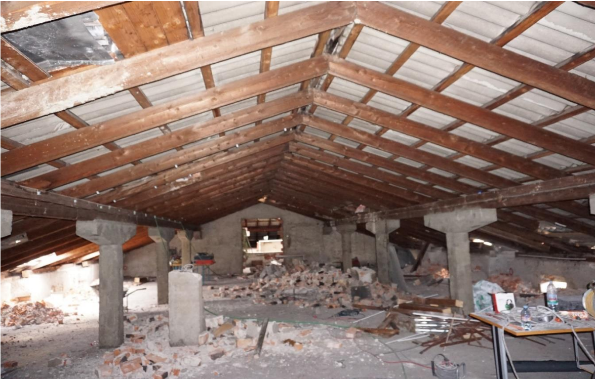
Figure 4-1: The roof of the faculty building prior to deconstruction.
