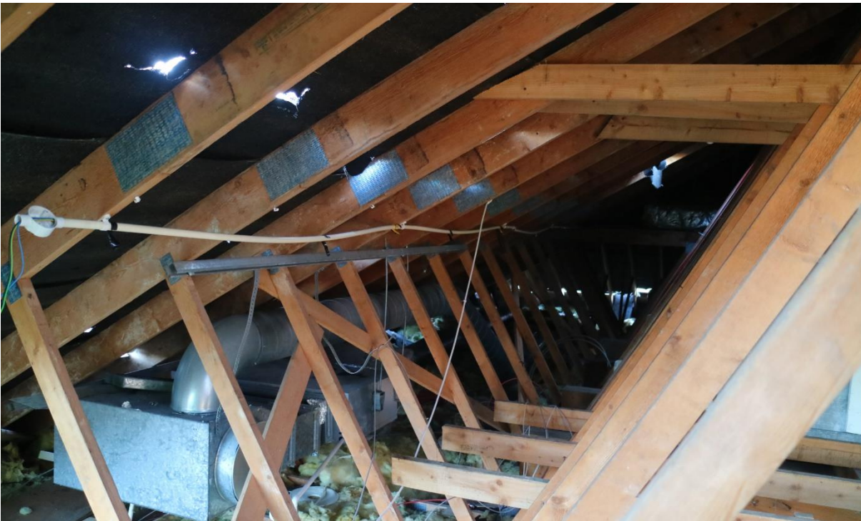
Figure 2-1: Roof trusses manufactured from spruce timber
