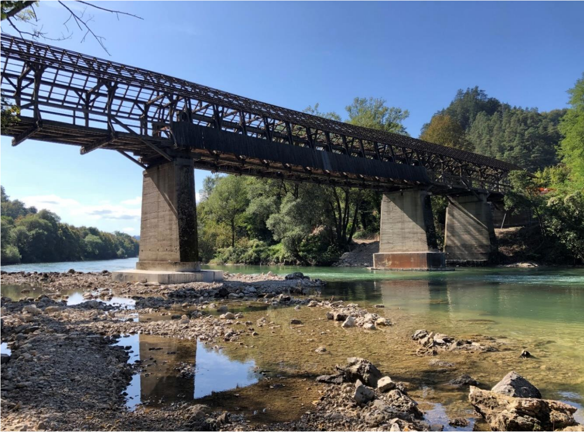
Figure 4-2: The bridge over the Sava river during deconstruction.
