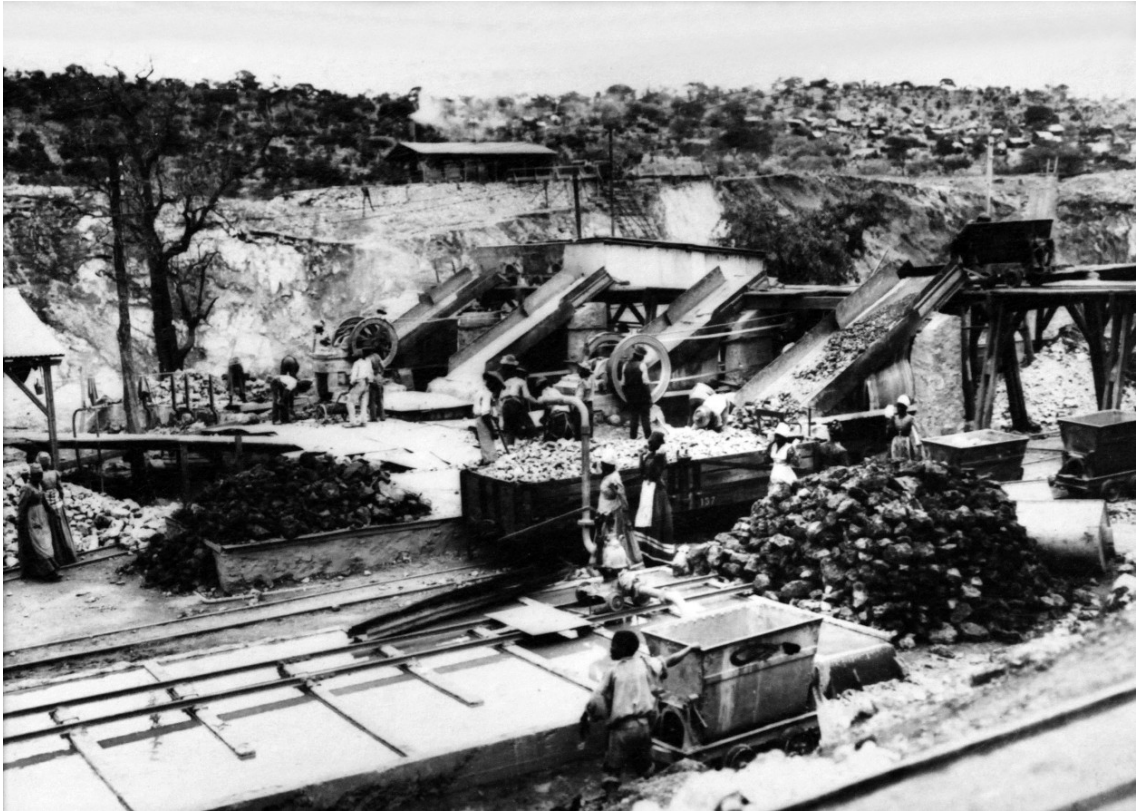
Figure 14: Women Sorting Ore for the Crusher, Tsumeb Mine
